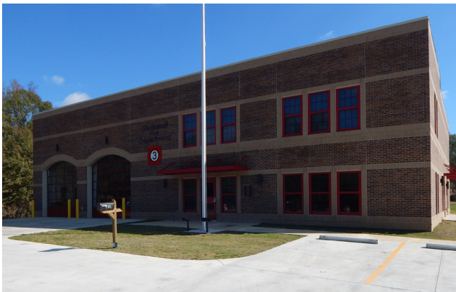
Gluckstadt Fire Department – Station #3, Yandell Road & Old Canton Road
