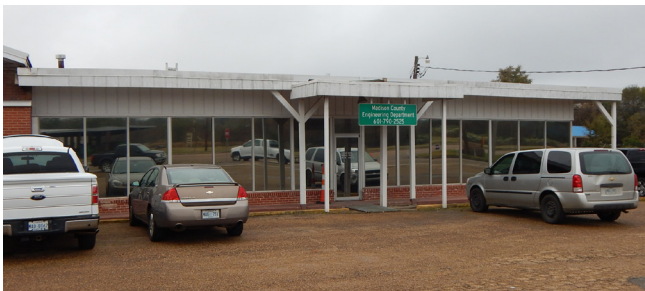
Engineering and Road Department
