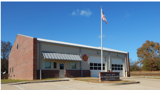
Valley View Fire Station
