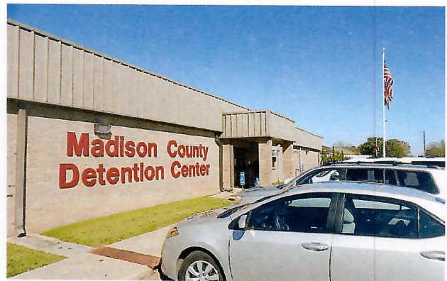
Madison County Detention Center
