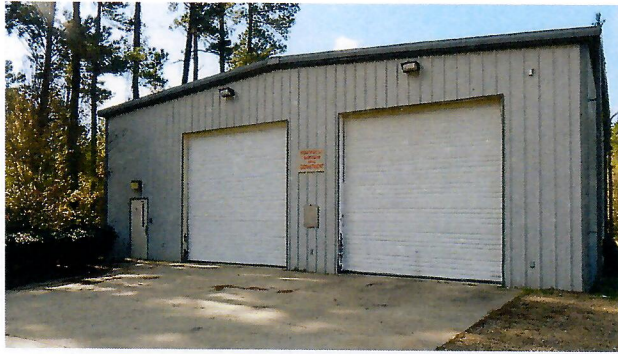
Southwest Fire Department, Station #1
