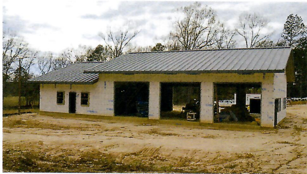
Southwest Fire Department, Station #2
