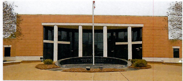
Circuit Court Building
