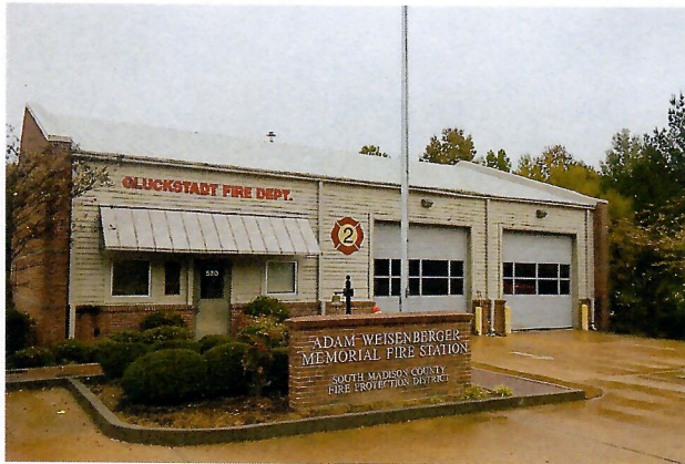
Gluckstadt Fire Department – Station #2, Stribling Road
