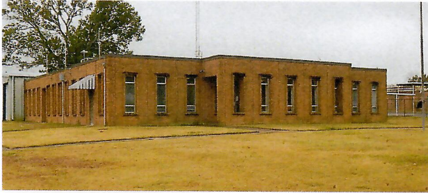
Madison County Emergency Services Complex
